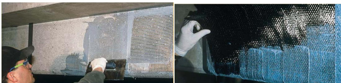
Figure 11: Hand lay-up dry system applied on a concrete girder [3]
